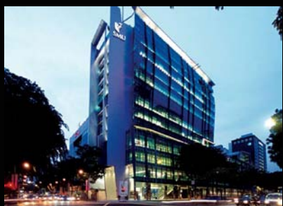
SMU Administration Bldg
